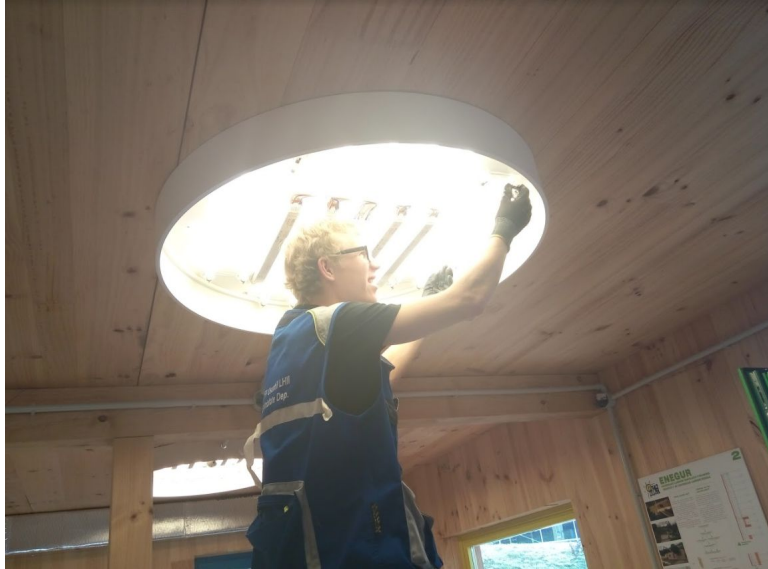
A photo that shows a student mounting DALI based LED illumination.
