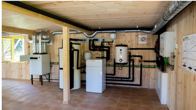
A inside view of the vent and thermal installations of ENEGUR
