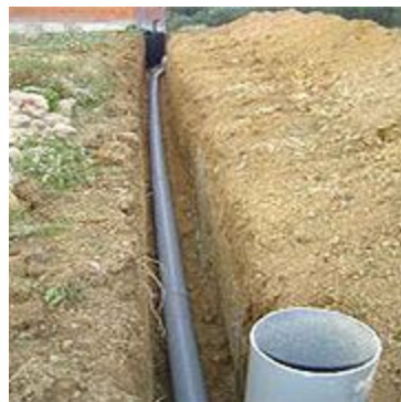
Canadian well installation
